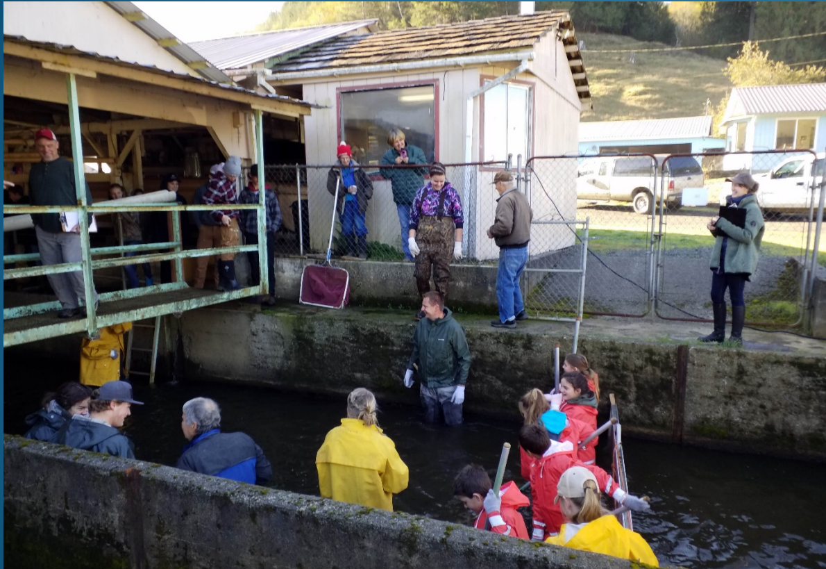
Repairs to concrete raceway
