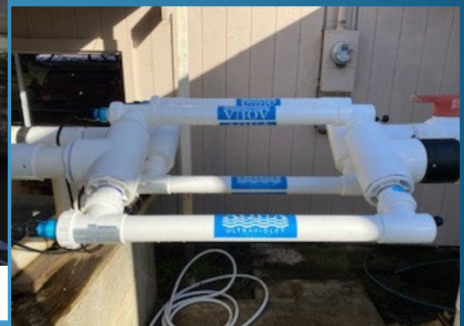
Electrical and Plumbing
